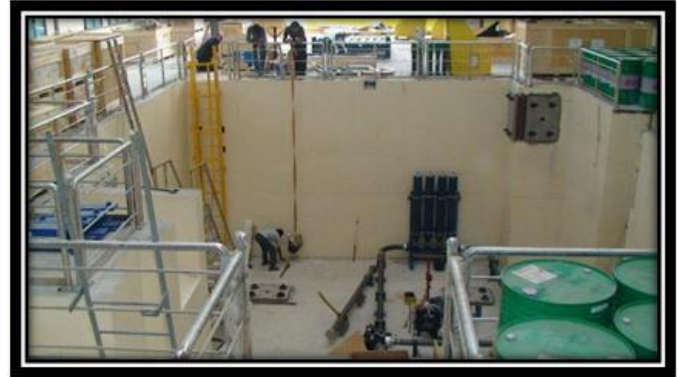
Fig. 11. Final stage before erection of shake table
