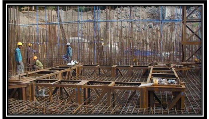
Fig. 8 Supporting steel structure
