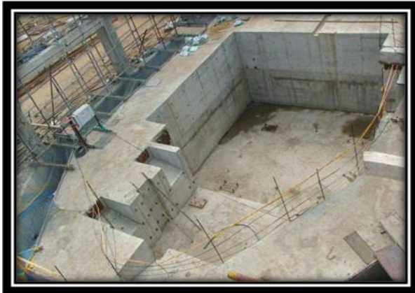
Fig. 9 Foundation block of shake table before erection
